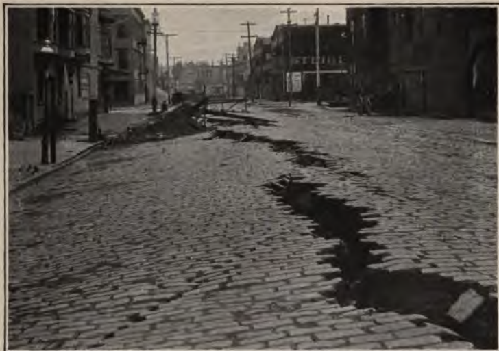
A. Gaping fissure in one of the streets of San Francisco from which the disturbed surface of the ground tilts outward.
